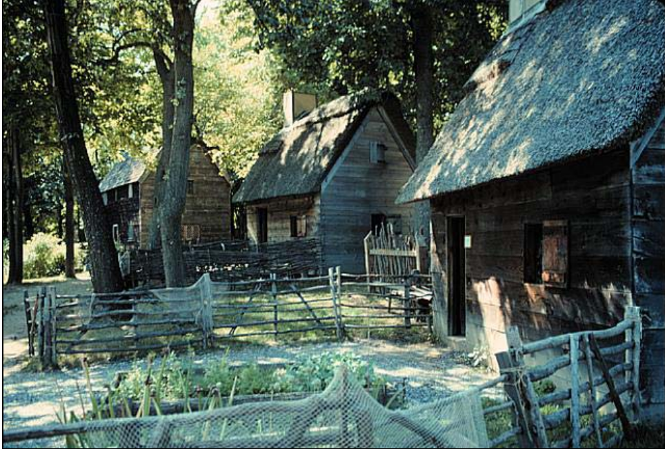
Pioneer Village Thatched Roofing
